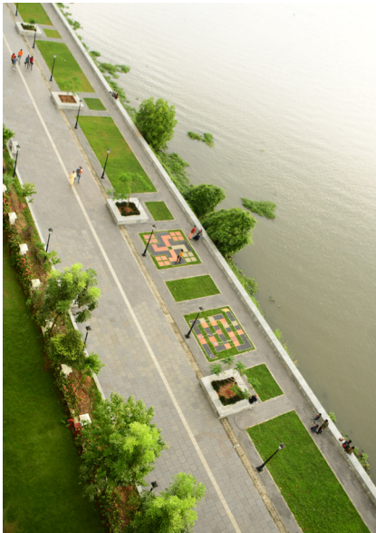
North end of Marine Drive walkway with inclusive activity spaces for all age groups
